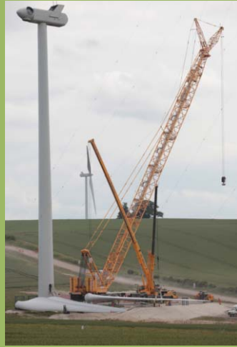
2. The hub and nacelle are put in place.
