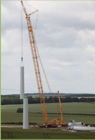
1. The tower sections are connected together.
